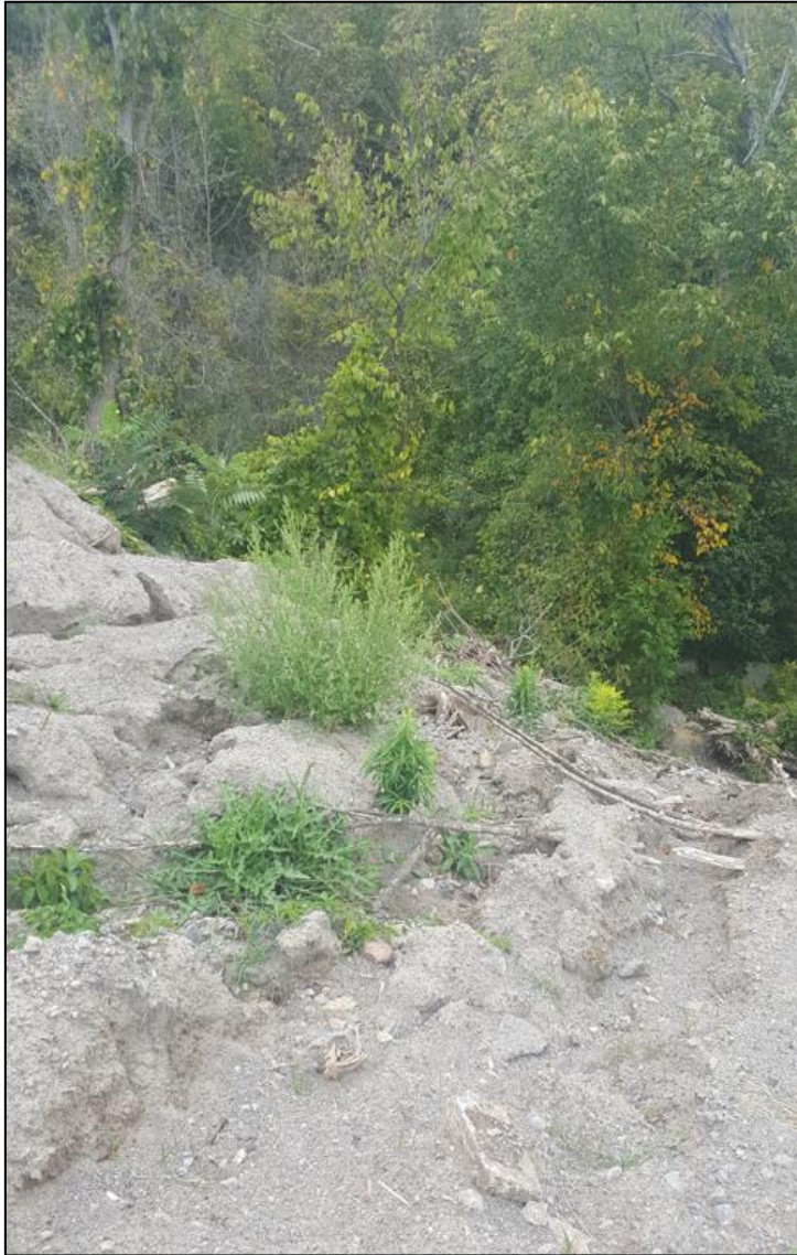
Photo 11: View of bare soil at the top of the slope where rills have formed in the soil as water drains over the slope to the SW, near BH102-21.
