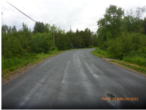
Figure 50 Images of Lynchs Rock Road Bridge F
