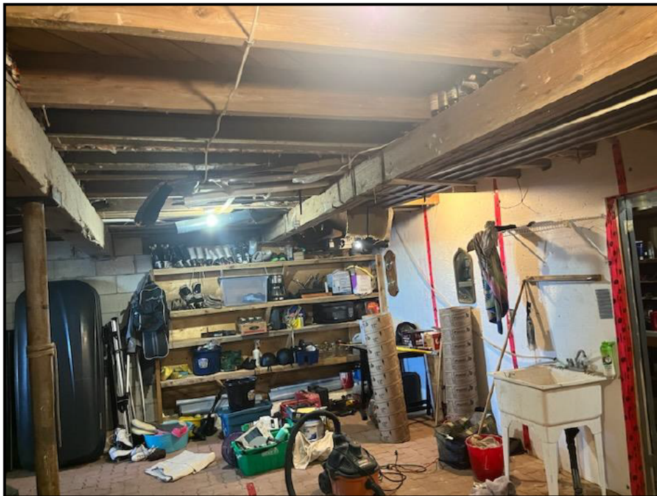
Photo 3 – Condition of Main Floor Framing
