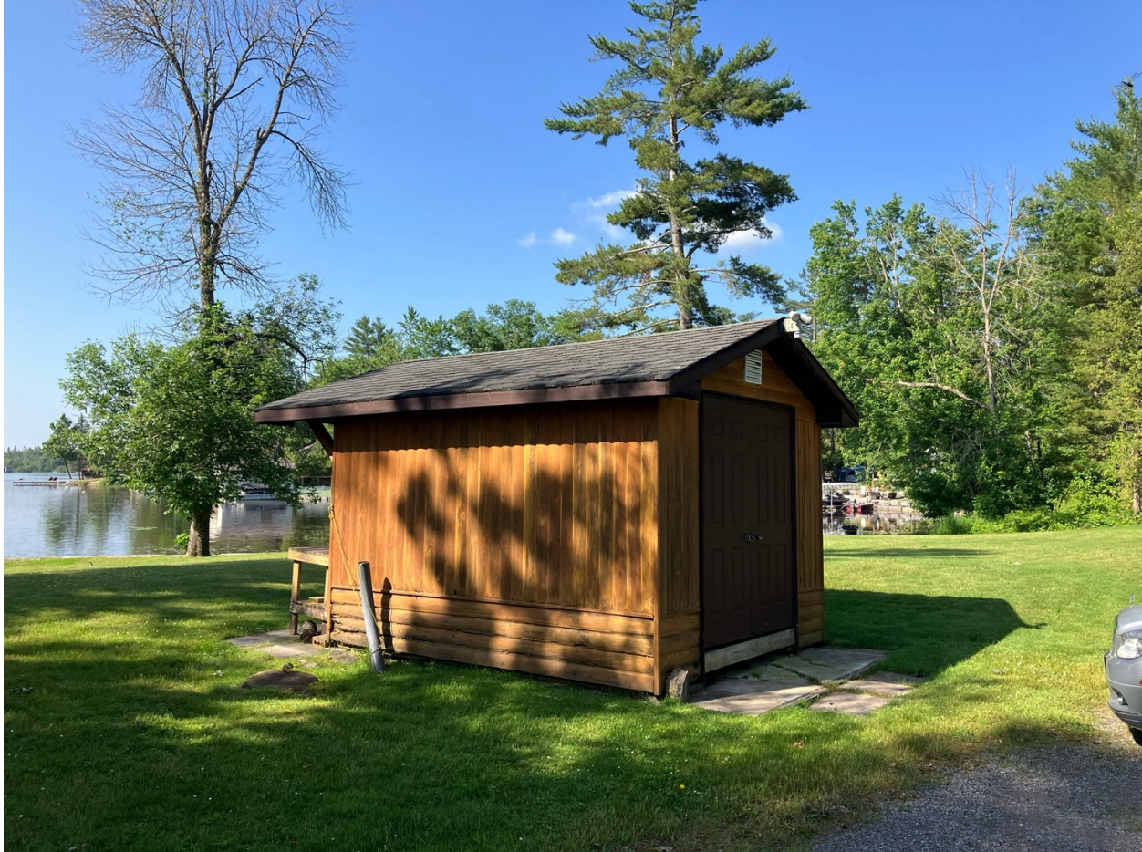
Figure 15: Existing wood frame shed (proposed to be demolished).
