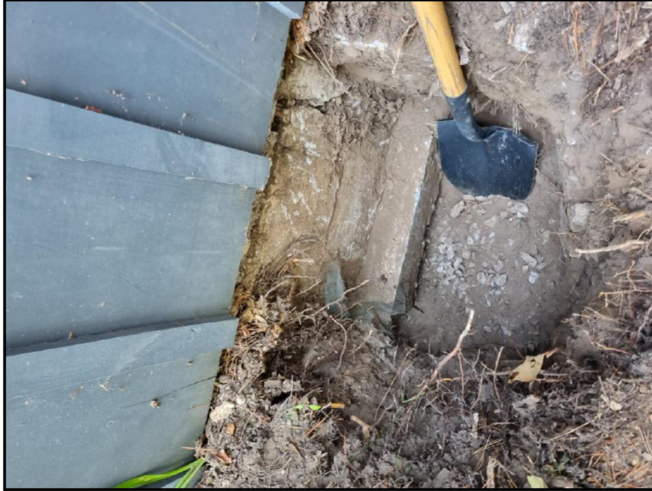
Photo 2 – Existing Non-frost Protected Foundation
